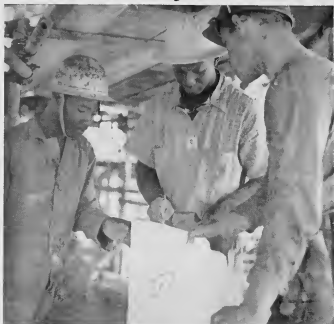
Installing Insulation, W. Young, G. Miller, and E. Diaz.
